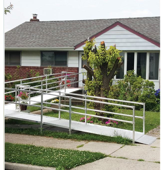
Handicapped ramp that was installed through the Town's Community Development Block Grant Program.
