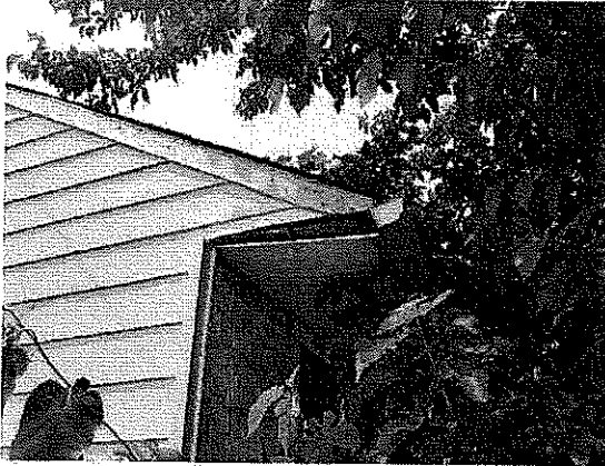
Corner (Northeast) – Overgrowth on building. Soffit collapsing. Missing / deteriorating siding.
