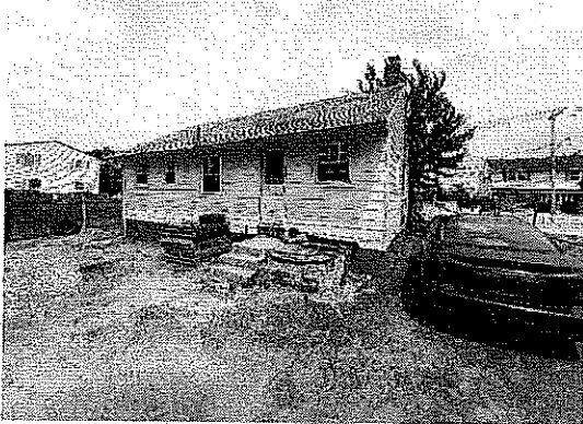
Rear Yard & Rear Façade (South) – Unsafe, dilapidated concrete patio. Unregistered car. Dangling wiring. Missing gutters. Roof dilapidated, shingles cracked.
