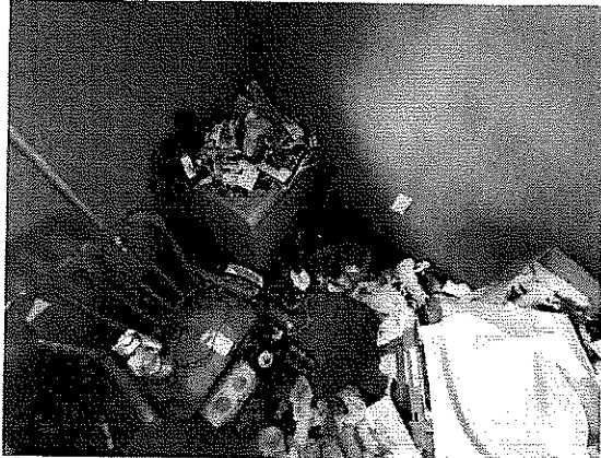
Bedroom (First Floor) – Personal items, trash, and debris strewn through interior. Evidence of transient activity.
