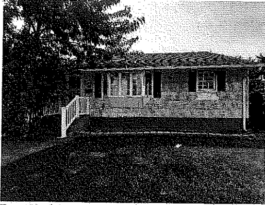
Front Yard & Front Façade (North) – Foundation cracked. Siding deteriorating. Roof dilapidated. Tree resting on building. Windows and doors not boarded.
