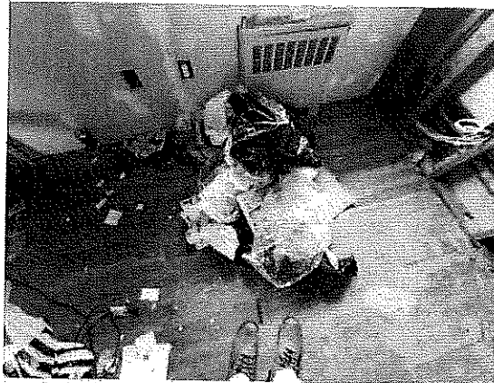
Interior (First Floor) – Trash and debris on floor. Unfinished electrical work and interior walls. Evidence of transient activity.
