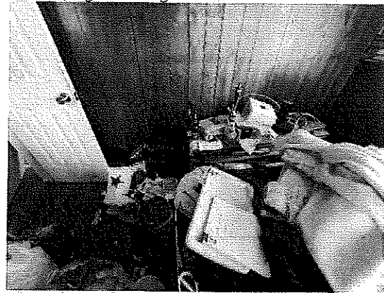
Living Room (First Floor) – Personal items, trash, and debris strewn through interior. Evidence of transient activity.
