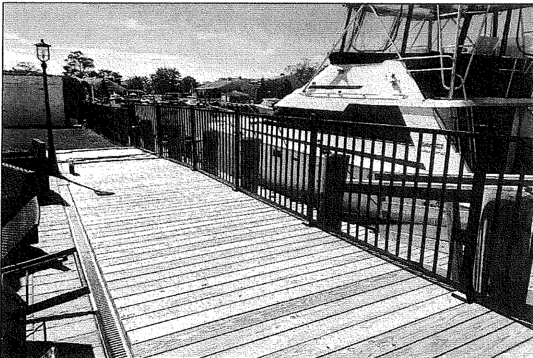
PHOTO 2: Overall view of backyard waterfront, looking southwest. Photo Date: 14 September 2022
